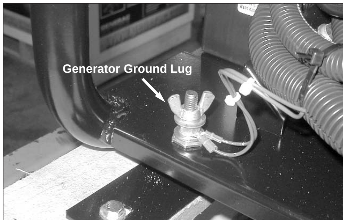
Figure 13 - Grounding the Generator
