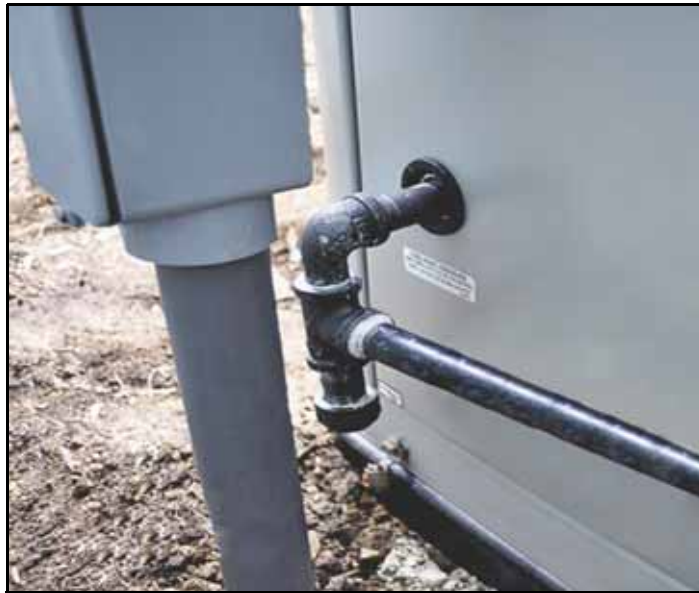
Figure 5-3. Sediment Trap (typical)
