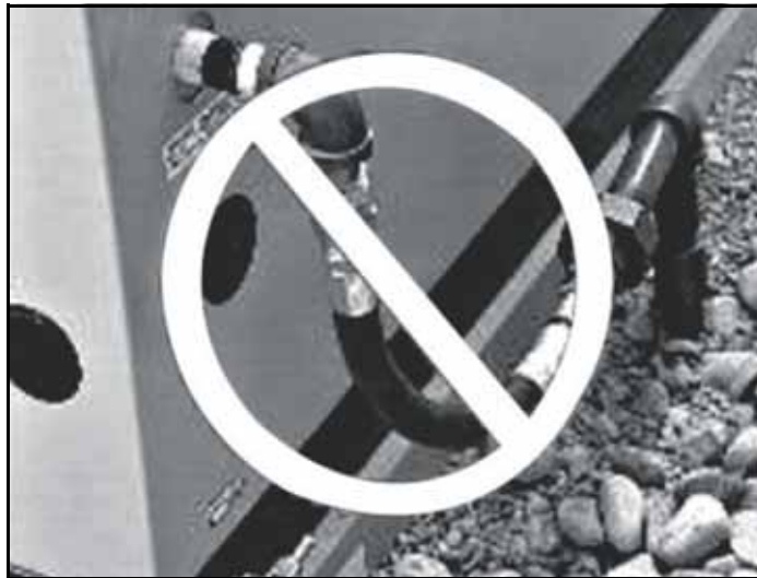
Figure 5-4. Incorrect Routing of Flexible Hose
