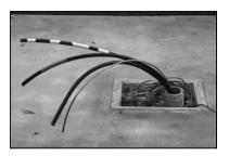
Regardless of configuration, power wiring, control wiring and wiring for the 15 or 20 Amp circuit required for the 2-Amp battery charger must always be in separate conduit.
