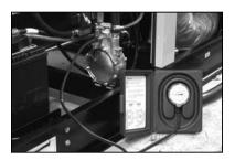
After checking all connections for leaks, check the static gas pressure at the secondary regulator to ensure there is sufficient pressure to operate the generator. (See Owner's Manual)
