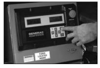
After shutting off the generator and restoring utility power, you'll need to set the current time and date and schedule the automatic exercise function in the generator control panel.
