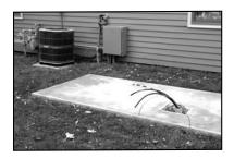
Position the electrical conduit for power wiring, control wiring and the battery charger circuit so the generator can be placed correctly on the pad.
