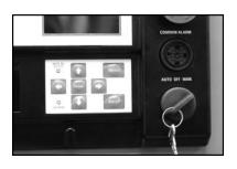
Select MANUAL on the generator control panel to start the generator with no loads present.
