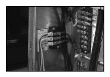
Connect the power leads for the battery charger to the 120-Volt, 15 or 20-Amp circuit as shown in the Installation Manual.
