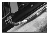
A section of UL or AGA approved flexible fuel line is required to protect the rigid fuel line connections against vibration from the generator.
