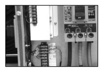
If phase rotation is incorrect, switch the A and C connections in the generator connection box and check phase rotation again. Refer to the Installation Manual for correct procedures.
