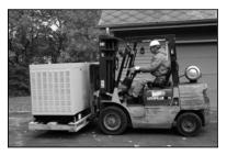
Use a forklift, boom truck or similar equipment with sufficient capacity to move the generator to the mounting pad area. The operator should be certified and experienced in generator installation.
