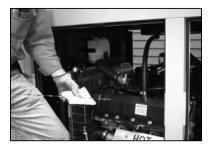
Before connecting the battery, make certain that normal utility voltage at the transfer switch is correct and the system is ready to be put into operation.
