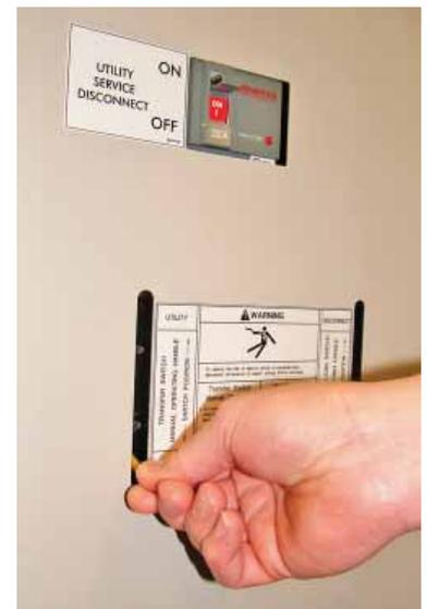
**NOTE:** Return handle to storage position in enclosure when finished with manual transfer.
