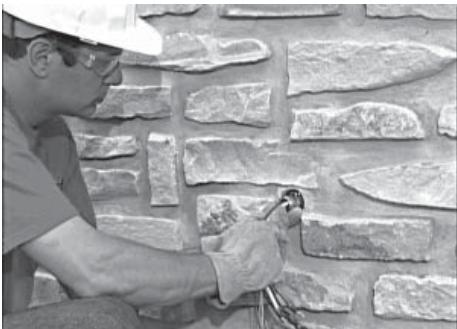
1. Drill a 1 3/4 inch hole and feed the conduit through the hole.
