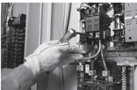
2. Connect the generator power leads to the E1 and E2 terminals on the transfer switch contactor.
