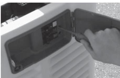
12. Connect the control wires to the correct terminals. The terminals are clearly marked N1, N2, 23 and 15B. If connecting a pre-wired switch a 0 (zero) wire will also be required.
