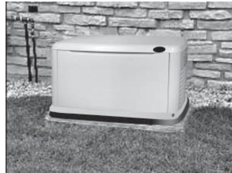
5. Set the generator onto the pad so that the gravel bed extends several inches beyond the generator on all sides. Make sure the generator is level within  $\frac{1}{2}$  inch.
