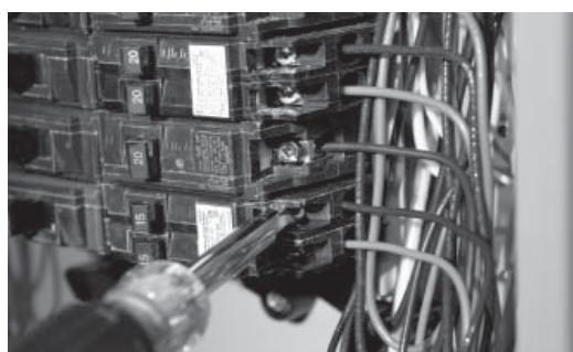
6. Next, connect the loads which are to be backed up. The breakers below the operator will be backed up by the generator during a power outage. Connect these loads to the appropriate sized breakers in the load center.
