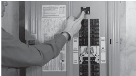
2. Switch the generator's main circuit breaker OFF and put the mode switch in the OFF position.
