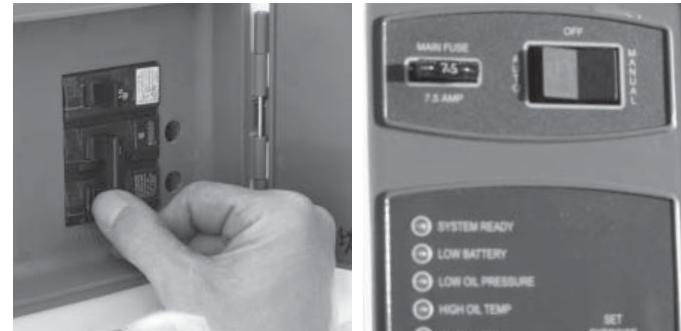
1. Switch the generator's main circuit breaker OFF and put the mode switch in the OFF position.
