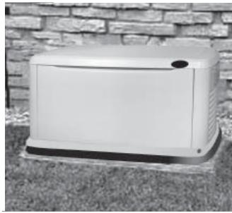
10. Shut OFF utility power and make sure the generator starts automatically.
