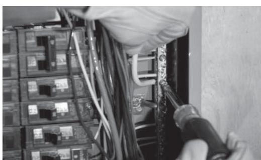
4. Connect the neutral wire from the utility and generator to the neutral bar on the right side of the load center panel and the generator equipment ground wire to the ground bar on the left side of the load center panel.
