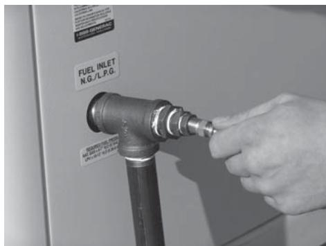
16. Unhook the gas meter and reinstall the port plug on the regulator.
