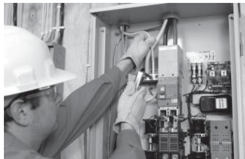
5. Neutral wires from the utility, generator and shedding panel are connected to the same neutral lug in the switch.
