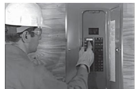
7. Make sure the 2-pole circuit breaker installed in the main distribution panel is in the OFF position.
