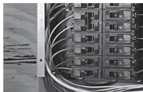
4. Each wire in the pre-wired transfer switch is color-coded to easily match circuits in the main panel to their new breakers in the transfer switch.
