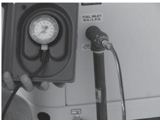
6. After checking for leaks, check the gas pressure at the T-fitting installed earlier to make sure there's enough pressure for proper generator operation. The local gas supplier is responsible for ensuring adequate pressure, so if the pressure is too low, or if it's greater than 14 inches of water column, contact the gas supplier.
