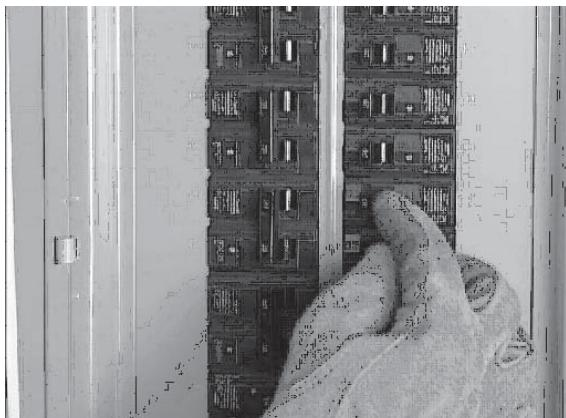
12. Shut OFF utility power again to automatically start the generator. When power has transferred to the generator, close each of the breakers in the distribution panel one at a time until the generator has accepted the entire load.
