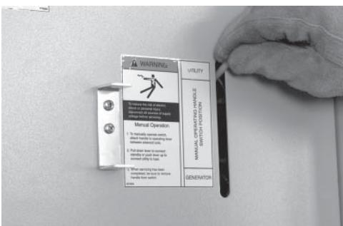
4. Locate the transfer handle and insert the metal end into the slot in the main contactor assembly. Pull the handle DOWN to move the main contacts to the standby power (generator) position.
