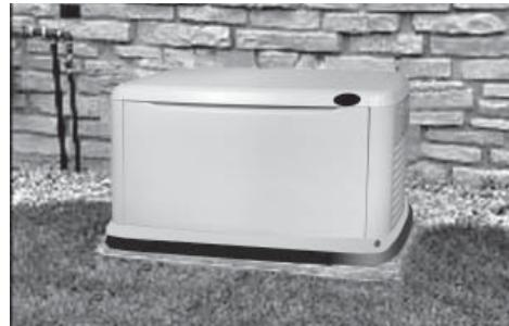
1. If the generator comes with an external connection box and 5' seal-tite whip pre-wired and connected to the generator, no additional connections are necessary at the generator. Skip the following section and proceed with Appendix A, RTS Pre-Wired Load Center Transfer Switch Installation & Operational Testing.
