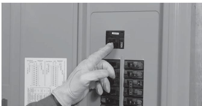
4. Make sure the central air conditioner will not start and simulate a power outage by shutting OFF utility power.
