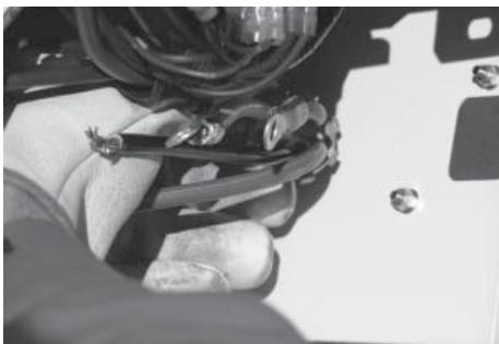
8. Remove the plastic plugs inside the main breaker access area to allow connection of the power leads to the circuit breaker.
