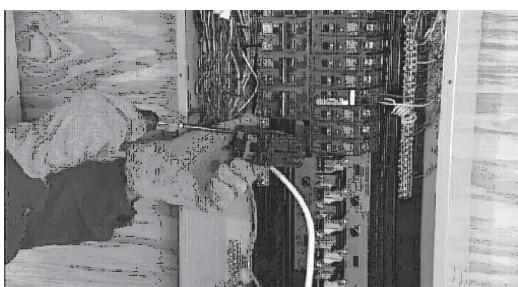
11. Install a 2-pole breaker in the distribution panel to protect the transfer switch. The required amp rating of the breaker depends on which transfer switch is used. If installing an 8-circuit, pre-wired load center switch, the breaker cannot exceed 40 Amps. For all other pre-wired load center switches the breaker cannot exceed 70 Amps. This breaker must be compatible with the existing electrical distribution panel.
