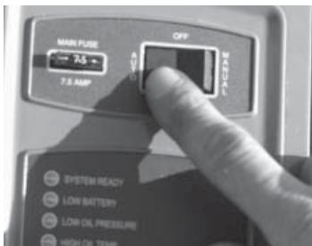
9. Now switch the generator's main breaker ON, and put the mode switch in AUTO.
