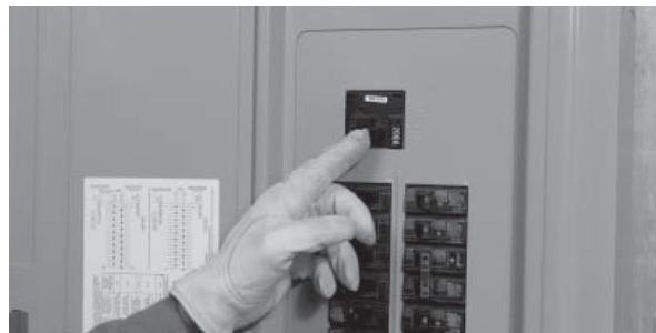
5. Make sure utility power is OFF and place all of the individual circuit breakers in the main distribution panel in the OFF position.
