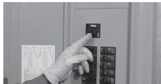
18. Shut OFF utility power again. The generator should start and the entire load should transfer to the generator. If the load is too large, the non-essential load shed switch will automatically shed the non-priority loads.
