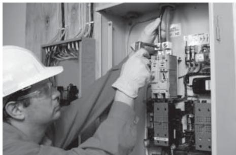
1. Connect the utility power leads from the meter to the Utility circuit breaker in the transfer switch.
