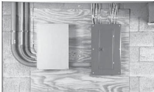
1. If installing the RTSE switch, the service was changed so make sure the terminations are good before re-energizing the utility.
