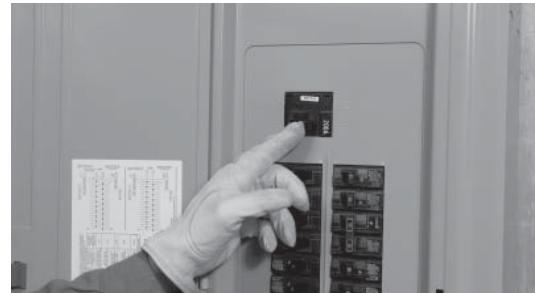
15. Shut OFF utility power again to automatically start the generator. When power on the lower half of the load center has transferred to the generator, turn ON each of the branch circuit breakers in the lower half of the load center, one at a time, until the generator has accepted the entire priority load.
