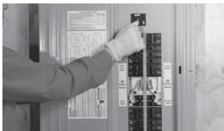
10. Switch ON the main utility breaker if not already on and switch on the utility supply breaker for the priority circuits. Make sure utility voltage at the load center is correct. Refer to NFPA 70E for the safety equipment required when working inside a live load center.
