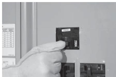
13. Shut OFF utility power at the main utility breaker and make sure the generator starts automatically.
