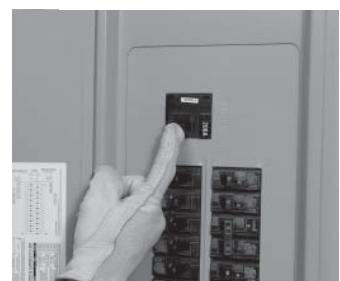
19. Close the main breaker to restore utility power and allow the engine to cool down and shut itself OFF.
