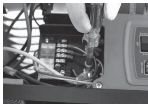
6. On 8 kW units, the main breaker is located inside the generator at the rear of the connection area.
