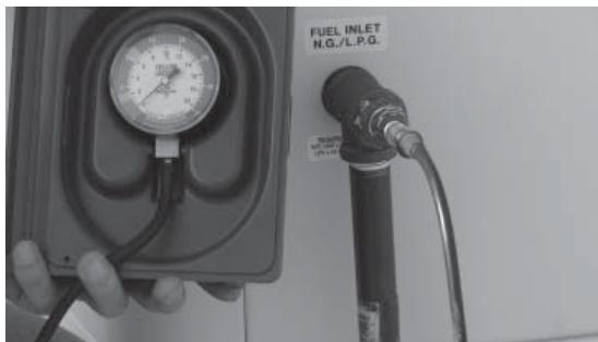
16. With the generator carrying the entire load, recheck gas pressure to verify that it's at the same level it was before the generator was started.
