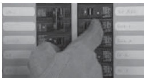
12. After the engine has completed its cool down cycle and shut down, shut OFF utility power again. When the generator is supplying power to the transfer switch, move the breakers in the switch to the ON position, one at a time, until the generator has accepted the entire priority load.
