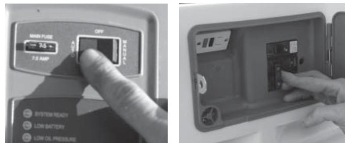
12. Switch the generator's main breaker ON and put the mode switch in AUTO.
