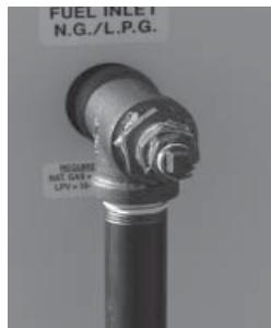
**NOTE:** Even if the generator is running smoothly at this point, a drop in gas pressure indicates that the supply is barely adequate to supply the generator's needs. Changes in the generator load, or additional gas demand by other appliances may affect the generator's performance. Verify gas pressure and pipe sizing. Unhook the manometer and reinstall the port plug.
