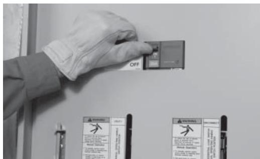
7. With all branch circuit breakers still OFF, close the main breaker by switching it to the ON position.
