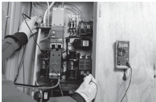
12. Check both line-to-line and line-to-neutral voltage on terminals E1 and E2. Terminations to T1 and T2 were made at the factory, but still make sure that voltage is correct at these terminals.
