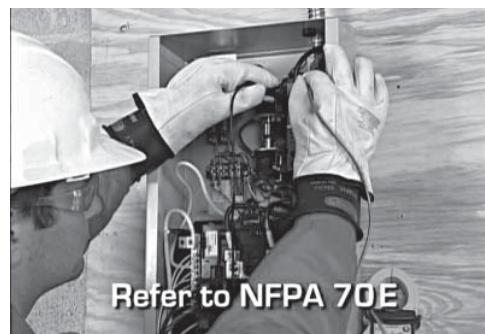
12. When all priority circuits have been moved to the transfer switch, close the main breaker to restore utility power and make sure utility voltage at the transfer switch is correct. Refer to NFPA 70-E for the safety equipment required when working inside a live transfer switch.
