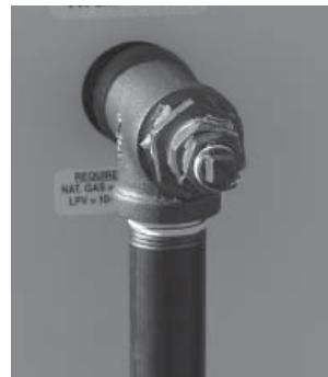
3. Where the gas line is to enter the generator, install a T-fitting to allow for gas pressure monitoring. On one opening of the fitting install a 1/4" NPT nipple and threaded plug. In some cases a sediment trap may also be installed.
