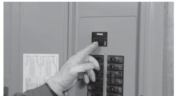
1. Switch the main breaker OFF. If there is a primary breaker in the sub-panel, make sure it is in the closed (ON) position.
