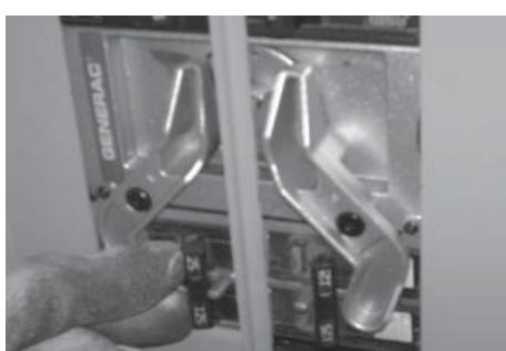
10. With utility power still OFF, switch the utility feed breaker (below the transfer operator on the left side of the load center) ON. This will also move the generator feed breaker to the OFF position.
