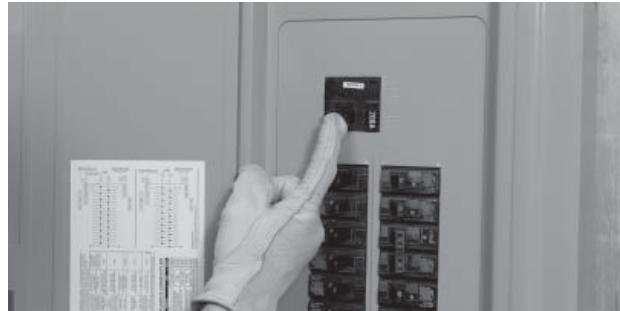
20. Close the main breaker to restore utility power and allow the engine to cool down and shut itself off.
