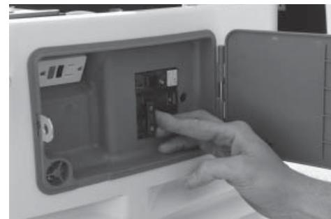
4. Manually switch the generator circuit breaker (just below the transfer operator) to the ON position. This will also move the utility feed circuit breaker to the OFF position.
