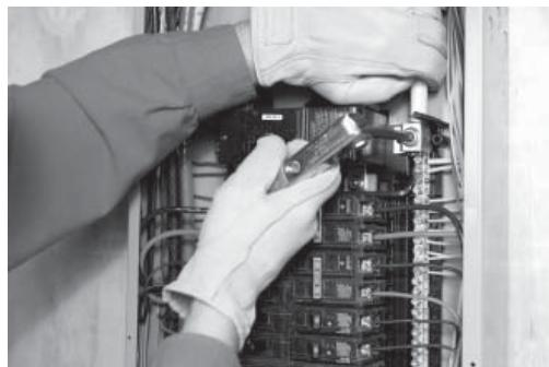
4. Be careful to support the lugs and torque the lugs in the transfer switch to the specifications shown in the transfer switch Owner's Manual.
