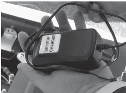
1. If the generator came with a separately packaged battery charger, it may be necessary to install the charger, either in the generator or in the transfer switch. Refer to documentation included with the battery charger for installation and wiring of the battery charger. For applications with RTSN, RTSE and GenReady transfer switches the charger needs to be mounted in the generator. Refer to documentation included with the battery charger for installation and wiring of the battery charger.
