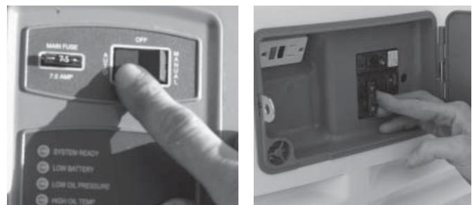
9. Switch the generator's main breaker to the ON position and put the mode switch in AUTO.
