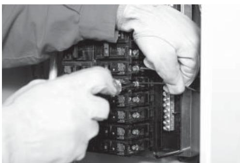
10. When three-conductor wiring is used, two 120 volt circuits will often share the same neutral wire. To avoid overloading the neutral, either move BOTH of the circuits that share the neutral or don't move either of them.
