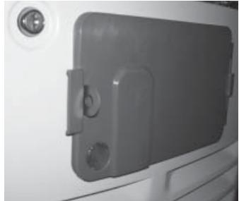
5. For 10-20 kW models, locate the metal hasp that is packaged in the owner's manual bag. Insert the hasp in the slot located on the left side of the external circuit breaker box. Be sure that the clip of the hasp is facing toward the front of the generator. If desired, lock the external box.
