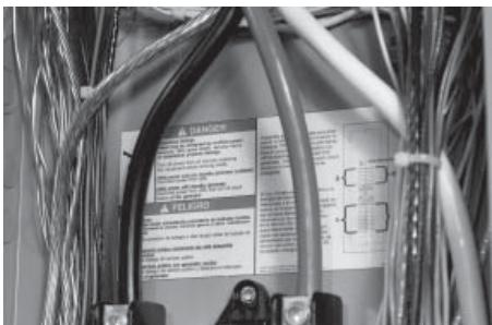
During installation, be careful to torque the lugs on all circuit breakers to the specifications listed in the load center Owner's Manual.
