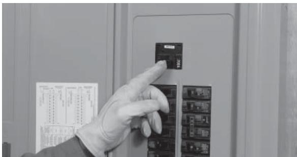
2. Switch the main utility breaker OFF. Refer to NFPA 70-E for the safety equipment required when working inside a live transfer switch.
