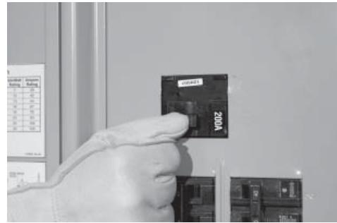
5. With the main breaker OFF, energize the utility and check the voltage at terminals N1 and N2 on the transfer contactor. If utility voltage is not approximately 240 volts, de-energize utility power and check all of the terminations between the utility and N1 and N2.
