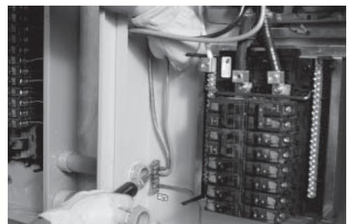
8. The grounding that is normally in the main panel must be accomplished in the Power Manager Load Shed transfer switch and must be disconnected in the existing distribution panel. Refer to the National Electrical Code (NEC) for complete information on grounding and bonding.
