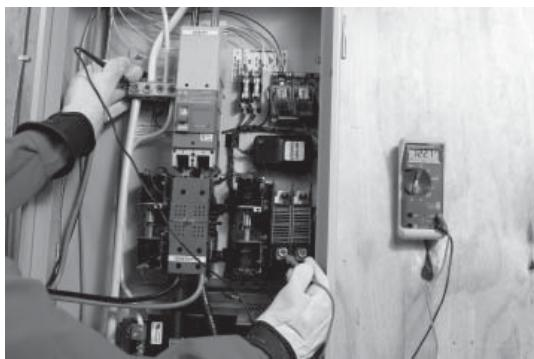
11. Next, check the voltage to the load shedding switch.
