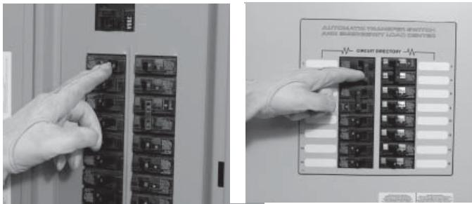
2. Next, make sure all of the individual circuit breakers in both the priority load center and in the non-priority sub-panel, are in the OFF position. If the sub-panel has a primary breaker, make sure it is in the OFF position as well.
