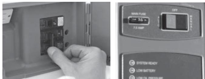
4. Switch the generator's main circuit breaker OFF and put the mode switch in the OFF position.
