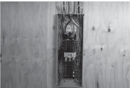
4. Protect against impact and mount the load center vertically to a rigid support structure. Make sure the load center is level and plumb.
