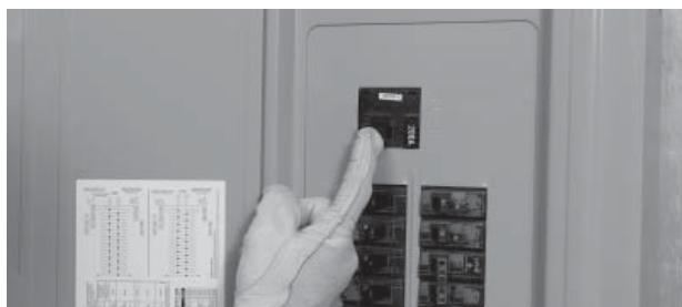
11. If everything worked properly, switch the main breaker to ON and make sure that power is automatically transferred back to the utility.
