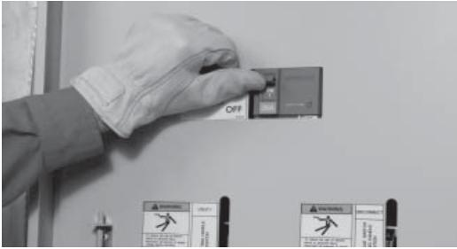
12. Switch the main breaker ON and make sure that power transfers back to the utility. The generator should shut down and go through a short cool-down cycle.
