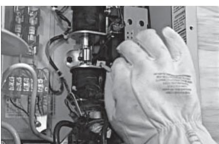
3. Locate the transfer handle, insert the metal end into the slot in the main contactor assembly and pull the handle DOWN to move the main contacts to the standby power, or generator position.
