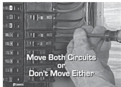
5. When three-conductor wiring is used, two 120 volt circuits will often share the same neutral wire. To avoid overloading the neutral, either move BOTH of the circuits that share the neutral or don't move either of them.
