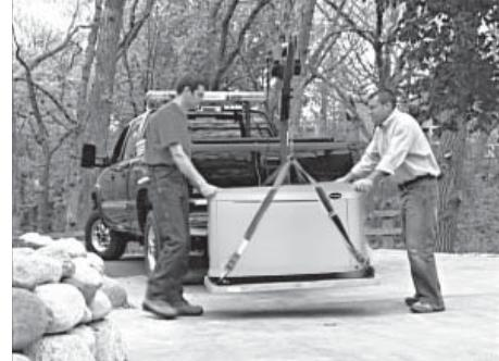
4. Make sure the lifting equipment to be used has sufficient capacity to safely handle the weight of the generator. Use nylon lifting straps and connect them to the lifting eyes on each corner of the base frame to avoid damaging the enclosure.
