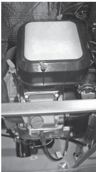
3. Where the gas line is to enter the generator, install a T-fitting to allow for gas pressure monitoring. On one opening of the fitting install a 1/4" NPT nipple and threaded plug. In some cases a sediment trap may also be installed.
