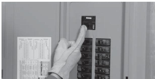
14. Switch the main breaker ON to restore utility power. The generator will continue to run to allow the engine to cool down before shutting itself off. Shut off utility power again. The generator should start and the entire priority load should transfer to the generator. Close the main breaker to restore utility power and allow the engine to cool down and shut itself off.
