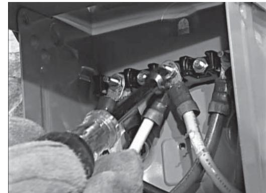
2. Remove the knockout in the back of the connection box, feed the wires through the back of the box and secure the conduit with the lock nut. Seal the hole with silicone caulk. Don't forget to caulk the hole inside the house as well.
