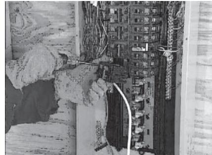
11. Install a 2-pole breaker in the distribution panel to protect the transfer switch. The required amp rating of the breaker depends on which transfer switch is used. Pre-wired load center switches the breaker cannot exceed 70 Amps. This breaker must be compatible with the existing electrical distribution panel.
