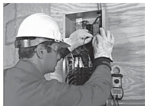
1. Switch the generator's main circuit breaker OFF and put the mode switch in the OFF position.
