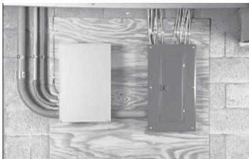
1. Before beginning any installation, make sure power is shut OFF to the main distribution panel and carefully read the Owner's Manual that came with the transfer switch. To simplify the installation process, the transfer switch should be mounted as close to the main distribution panel as possible. Make sure no water or corrosive substances can drip onto the transfer switch enclosure.
