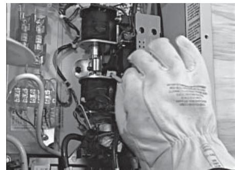
3. Locate the transfer handle, insert the metal end into the slot in the main contactor assembly and pull the handle DOWN to move the main contacts to the standby power, or generator position.
