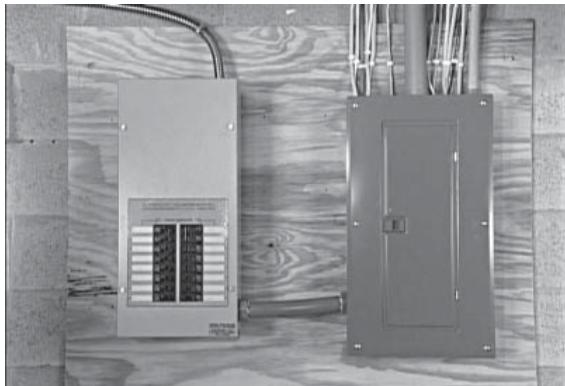
1. Before beginning any installation, make sure power is shut OFF to the main distribution panel and carefully read the Owner's Manual that came with the transfer switch. The distributed load center switch must be mounted close enough to the main distribution panel to accommodate the two-foot, pre-wired conduit. Make sure no water or corrosive substances can drip onto the transfer switch enclosure.
