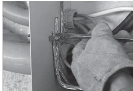
4. Complete the transfer switch wiring by connecting the equipment ground wires from both the utility and the generator to the ground lug.
