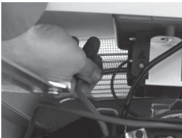
8. Now connect the red and black power leads to the circuit breaker. Since this is a single-phase application, it doesn't matter which wire is connected to which lug.
