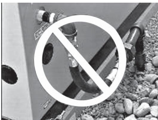
5. Never bend the flexible fuel line to avoid using an elbow. Bending the flexible line decreases its ability to absorb vibrations and defeats its purpose as well as constricts the actual fuel flow.
