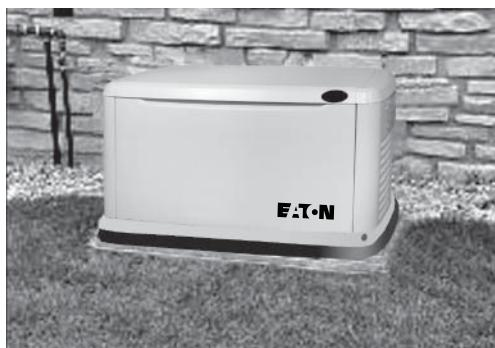
5. Set the generator onto the pad so that the gravel bed extends several inches beyond the generator on all sides. Make sure the generator is level within  $\frac{1}{2}$  inch.
