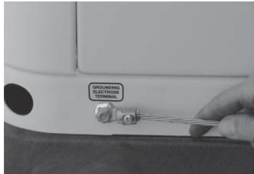
6. Connect an approved ground strap to the grounding lug on the base frame and to an approved earth ground or grounding rod as specified by local regulations.
