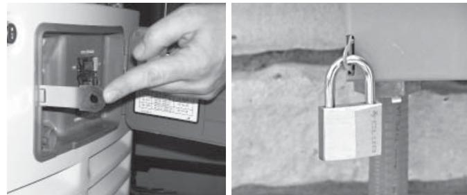
5. For 10-20 kW models, locate the metal hasp that is packaged in the owner's manual bag. Insert the hasp in the slot located on the left side of the external circuit breaker box. Be sure that the clip of the hasp is facing toward the front of the generator. If desired, lock the external box.
