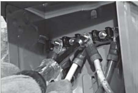
3. Mount the connection box (if used) so that it completely covers the hole in the wall. Caulk around the sides and top of the box to ensure a good seal.
