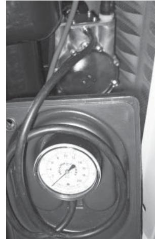
6. After checking for leaks, check the gas pressure at the T-fitting installed earlier to make sure there's enough pressure for proper generator operation. The local gas supplier is responsible for ensuring adequate pressure, so if the pressure is too low, or if it's greater than 14 inches of water column, contact the gas supplier.
