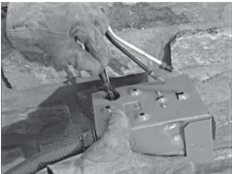
2. Remove the knockout in the back of the connection box (if used), feed the wires through the back of the box and secure the conduit with the lock nut.
