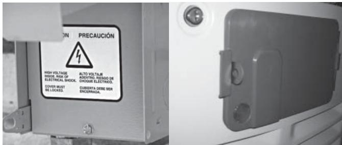
4. Replace the protective cover plate and retaining screw, and lock the connection box.
