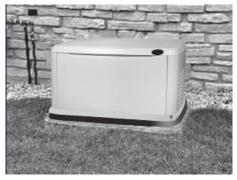
5. Set the generator onto the pad so that the gravel bed extends several inches beyond the generator on all sides.
