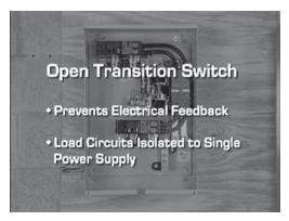
6. The transfer switch being used is an open transition switch. Open transition switches prevent electrical feedback between the generator and the utility by only allowing load circuits to be connected to one power supply at a time.
