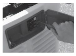
5. Remove the plastic plugs inside the main breaker access area to allow connection of the power leads to the circuit breaker.
