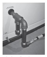
4. When connecting the gas line to the generator, use the provided section of UL Listed or AGA-approved flexible fuel line in accordance with local regulations. The purpose of the flexible fuel line is to ensure that vibration from the generator does not cause a gas leak at one of the connection points, so it's important that the line be installed with as few bends as possible.
