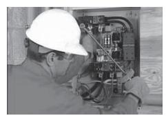
Being careful to support the lugs, torque the lugs in the transfer switch to the specifications shown on the transfer switch. Decal located on the inside of the switch door.
