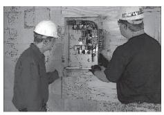
Protect against impact and mount the switch vertically to a rigid support structure. Make sure the switch is level and plumb. Check local codes before wiring the transfer switch. Some jurisdictions require that wiring inside the switch be done by a licensed electrician.
