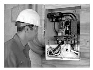
3. The grounding that is normally in the main panel must be accomplished in the service rated switch and must be disconnected in the existing distribution panel. Refer to the National Electrical Code (NEC) for complete information on grounding and bonding.
