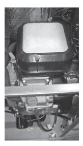
3. Where the gas line is to enter the generator, install a T-fitting to allow for gas pressure monitoring. In some cases a sediment trap may also be installed.
