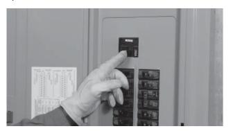
13. Shut OFF utility power and make sure the generator starts automatically after the line interrupt delay.
