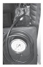
6. After checking for leaks, check the gas pressure at the regulator ports inside the generator to make sure there's enough pressure for proper generator operation.
