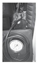
16. With the generator carrying the entire load, recheck gas pressure to verify that it's at the same level it was before the generator was started.
