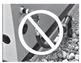
Never bend the flexible fuel line to avoid using an elbow.
