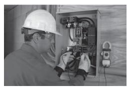
8. Check to be sure that voltage and frequency from the generator is correct. If line-to-line voltage is not approximately 240 volts, refer to the generator Owner's Manual for the proper adjustment procedures. If line-to-neutral voltage is not approximately 120 volts, check the neutral connection between the generator and transfer switch.
