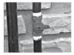
2. Most applications will require an external manual shutoff valve on the fuel line.
