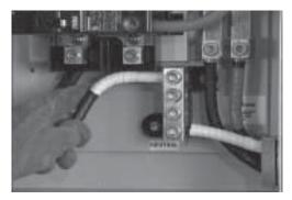
2. Neutral wires from both the utility and the generator are connected to the same neutral lug in the switch.
