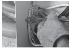
4. Complete the transfer switch wiring by connecting the equipment ground wires from both the utility and the generator to the ground lug.
