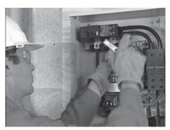
1. Connect the power leads from both the generator and the utility to the appropriate lugs in the transfer switch. The lugs are clearly marked in the switch.
