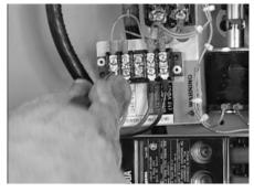
3. Connect the control wires from the generator to the designated locations. Wires 0, 23 and 194 connect to the terminal strip; N1, N2, and T1 connect directly to the fuse holders.
