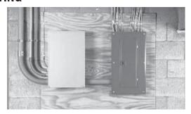
Before beginning any installation, make sure power is shut OFF to the main distribution panel and carefully read the Owner's Manual that came with the transfer switch. To simplify the installation process, the transfer switch should be mounted as close to the main distribution panel as possible. Make sure no water or corrosive substances can drip onto the transfer switch enclosure.
