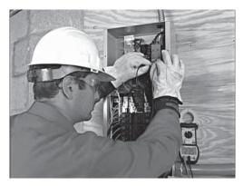
Energize the utility and check line-to-line and line-to-neutral voltage at terminals N1 and N2 on the transfer contactor. If line-to-line voltage is not approximately 240 volts, de-energize utility power and check the terminations between the utility and N1 and N2.
