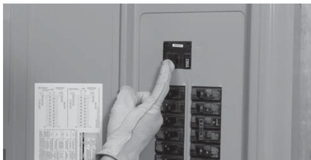
20. Close the main breaker to restore utility power and allow the engine to cool down and shut itself off.
