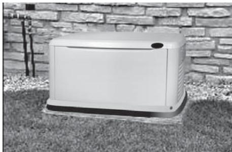
18. The generator will continue to run to allow the engine to cool down, then shut itself off.
