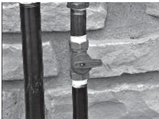
7. When finished checking the gas pressure, close the manual shutoff valve.
