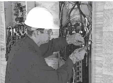
9. Make sure each circuit moved is protected by the same size breaker in the transfer switch. 15 Amp circuits must be connected to 15 Amp breakers and 20 Amp circuits to 20 Amp breakers.
