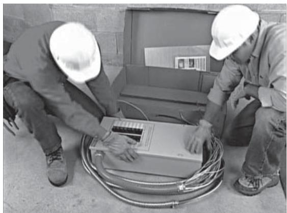
2. Always inspect the switch for shipping damage. Never mount a transfer switch that shows any evidence of damage.
