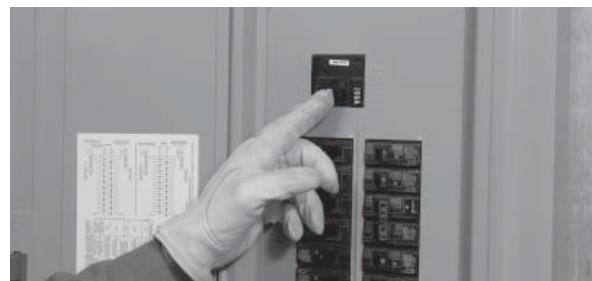
15. Shut OFF utility power again to automatically start the generator. When power has transferred to the generator, close each of the breakers in the distribution panel one at a time until the generator has accepted the entire load.
