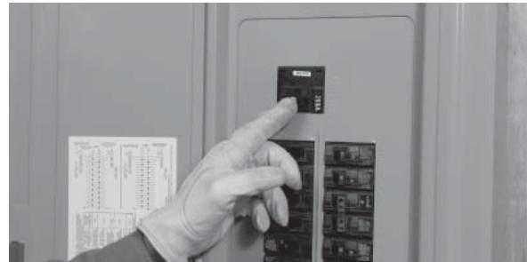
13. Shut OFF utility power and make sure the generator starts automatically after the line interrupt delay.
