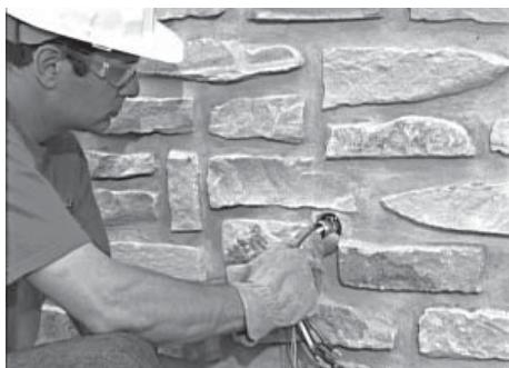
1. Drill a 1 3/4 inch hole and feed the conduit through the hole.
