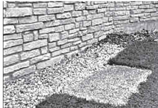
2. Place the unit so air vents won't become clogged with leaves, grass, snow or debris. Make sure exhaust fumes will not enter the building through eaves, windows, ventilation fans or other air intakes. Dig a rectangular area approximately five inches deep and about six inches longer and wider than the footprint of the generator. Cover with polyurethane film and fill with pea gravel or crushed stone. Compact and level the stone. A concrete pad can be poured if desired.
