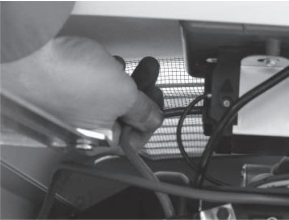
6. Now connect the power leads to the circuit breaker. Since this is a single-phase application, it doesn't matter which power lead is connected to which lug.
