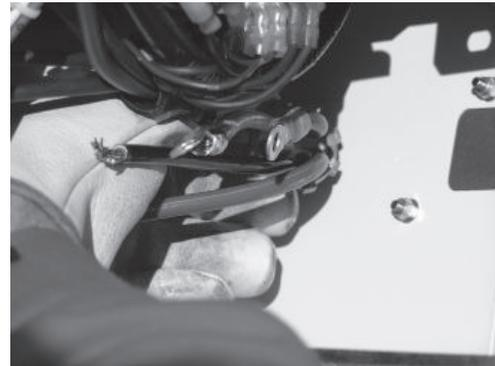
2. Feed the wires through the back of the generator and secure the conduit.
