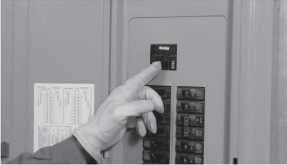
1. Switch the main utility breaker OFF. Refer to NFPA 70-E for the safety equipment required when working inside a live transfer switch.
