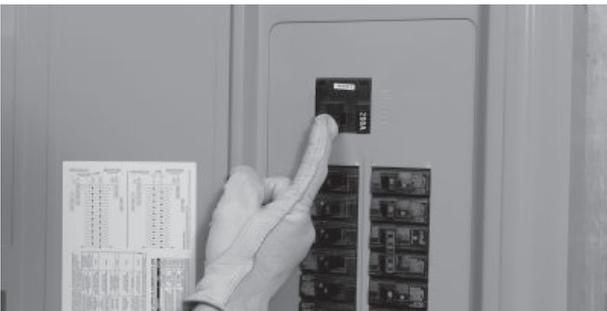
19. Close the main breaker to restore utility power and allow the engine to cool down and shut itself off. Operational tests are now complete. Refer to Appendix B – Setting the Automatic Exercise Function to complete the installation.
