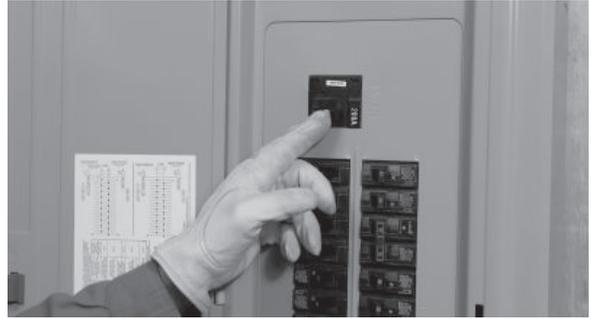
4. Make sure utility power is OFF and place all of the individual circuit breakers in the main distribution panel in the OFF position.
