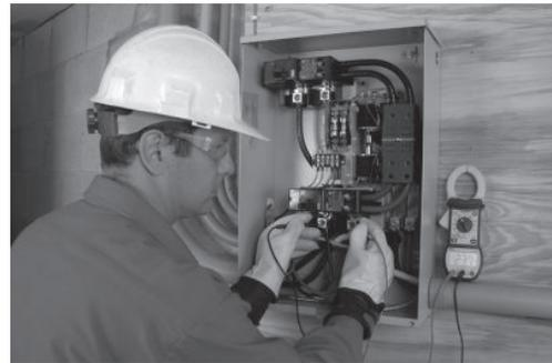
7. Check to be sure that voltage and frequency from the generator is correct. If line-to-line voltage is not approximately 220 volts, refer to the generator Owner's Manual for the proper adjustment procedures. If line-to-neutral (if applicable) voltage is not approximately 110 volts, check the neutral connection between the generator and transfer switch.
