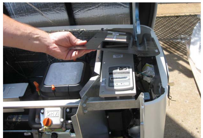
Figure 1 — Remove Control Panel Cover
