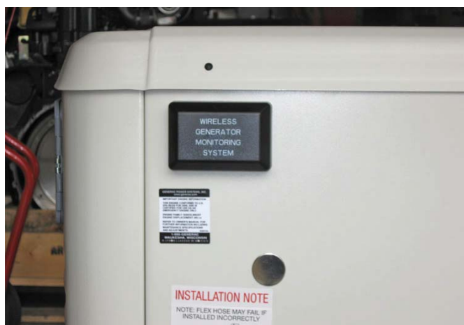
Figure 3 — Mount Transceiver
