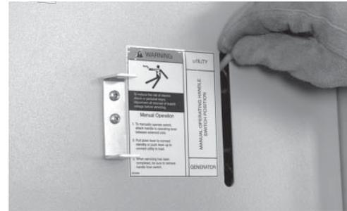
10. With utility power still OFF, use the transfer handle to move the main contacts to the UP (utility) position.
