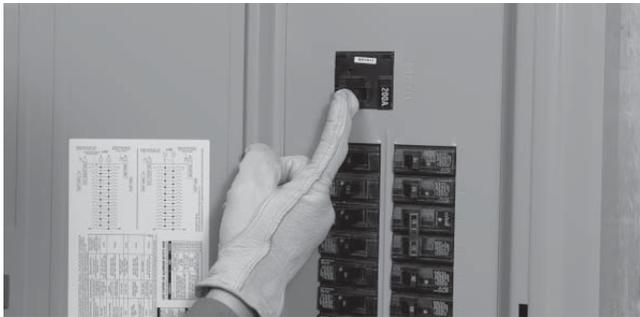
14. Switch the utility breaker to ON and make sure that power is automatically transferred back to the utility.
