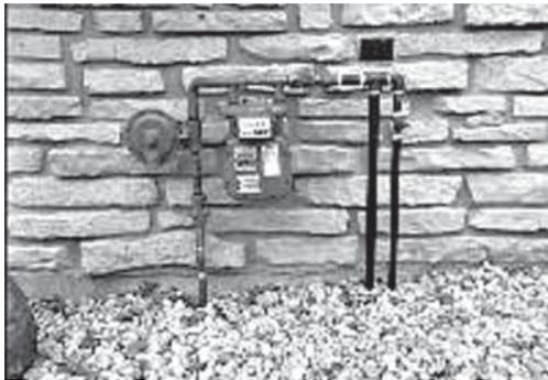
1. Both natural gas and LP Vapor are highly volatile substances, so strict adherence to all safety procedures, codes, standards and regulations is essential. Gas line connections should be made by a certified plumber familiar with local codes. Always use AGA-approved gas pipe and a quality pipe sealant or joint compound. Verify the capacity of the natural gas meter or the LP tank in regards to providing sufficient fuel for both the generator and other operating appliances.
