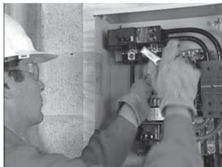
1. Connect the power leads from both the generator and the utility to the appropriate lugs in the transfer switch. The lugs are clearly marked in the switch.
