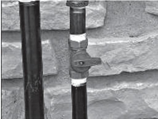
6. When finished checking the gas pressure, close the manual shutoff valve.
