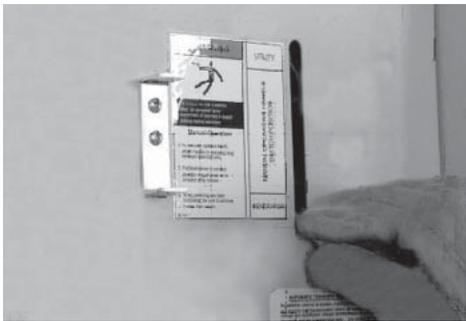
6. Locate the transfer handle, insert the metal end into the slot in the main contactor assembly. Pull the handle DOWN to move the main contacts to the standby power (generator) position. NEVER OPERATE THE TRANSFER SWITCH MANUALLY WHEN LOADS ARE CONNECTED.
