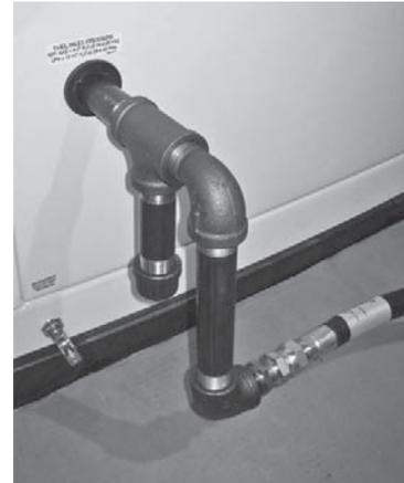
3. When connecting the gas line to the generator, use the provided section of UL Listed or AGA-approved flexible fuel line in accordance with local regulations. The purpose of the flexible fuel line is to ensure that vibration from the generator does not cause a gas leak at one of the connection points, so it’s important that the line be installed with as few bends as possible. Installing a sediment trap is also recommended.
