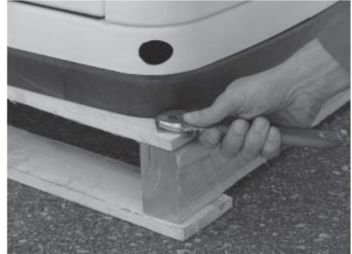
3. Inspect the generator for shipping damage and if necessary, file a claim with the shipper. Remove the bands holding the generator to the wooden pallet.
