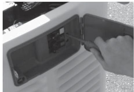
5. Remove the plastic plugs inside the main breaker access area to allow connection of the power leads to the circuit breaker.
