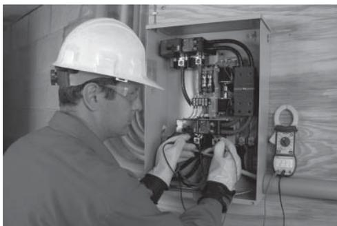
8. Check to be sure that voltage and frequency from the generator is correct. If line-to-line voltage is not approximately 240 volts, refer to the generator Owner's Manual for the proper adjustment procedures. If line-to-neutral voltage is not approximately 120 volts, check the neutral connection between the generator and transfer switch.
