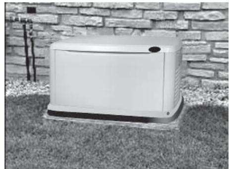
5. Set the generator onto the pad so that the gravel bed extends beyond the generator on all sides. Make sure the generator is level within 1/2 inch.
