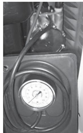
5. After checking for leaks, check the gas pressure at the regulator ports inside the generator to make sure there's enough pressure for proper generator operation. The local gas supplier is responsible for ensuring adequate pressure, so if the pressure is too low, or if it's greater than 14 inches of water column, contact the gas supplier.
