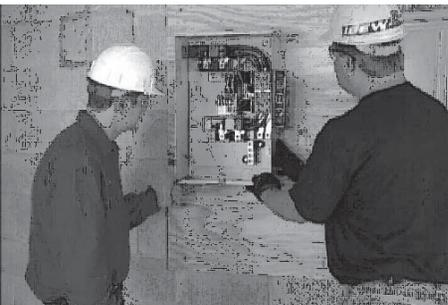
3. Protect against impact and mount the switch vertically to a rigid support structure. Make sure the switch is level and plumb. Check local codes before wiring the transfer switch. Some jurisdictions require that wiring inside the switch be done by a licensed electrician.
