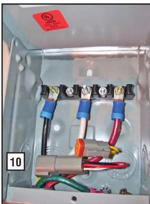
10. Lift cover. Remove internal cover plate screw and internal cover. Remove the knock out in the lower right corner of the external connection box. From the rear of the connection box, feed wires, 4-pin and 2-pin plugs into box. Slip the lock nut over wires and plugs and tighten securely onto conduit coupling. Using appropriate fasteners, mount external connection box over pre-drilled
