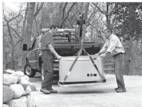
4. Make sure the lifting equipment to be used has sufficient capacity to safely handle the weight of the generator.
