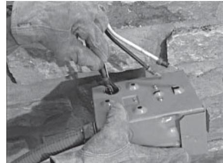
5. After checking for leaks, check the gas pressure at the REGULATOR to make sure there's enough gas pressure for generator operation. See Owner's Manual for fuel pressure specifications. If not within these limits, contact your local gas supplier.
