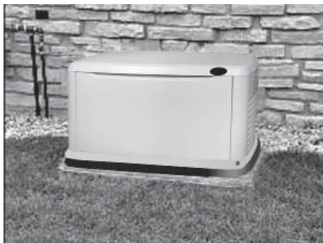
5. Set the generator onto the pad so that the gravel bed extends beyond the generator on all sides.
