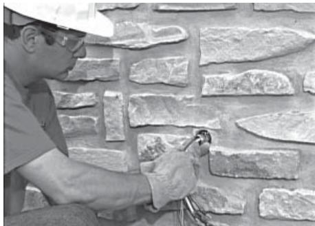
1. Drill the appropriate size hole and feed the conduit through the hole.
