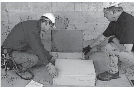
2. Always inspect the switch for shipping damage. Never mount a transfer switch that shows any evidence of damage.
