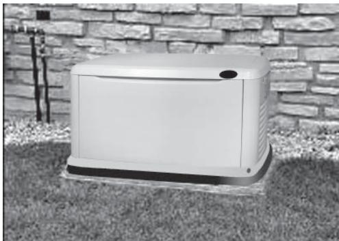
1. Locate the mounting area as close as possible to the transfer switch and fuel supply.
