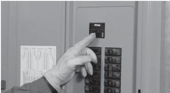
5. Make sure utility power is OFF and place all of the individual circuit breakers in the main distribution panel in the OFF position.
