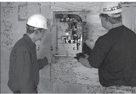
3. Protect against impact and mount the switch vertically to a rigid support structure. Make sure the switch is level and plumb. Check local codes before wiring the transfer switch. Some jurisdictions require that wiring inside the switch be done by a licensed electrician.
