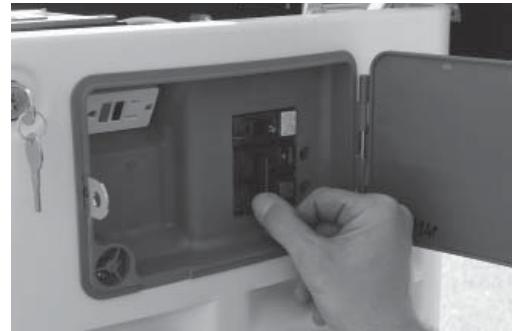
9. Switch the generator's main circuit breaker OFF and put the mode switch in the OFF position to shut down the generator.
