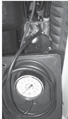
16. With the generator carrying the entire load, recheck gas pressure to verify that it's at the same level it was before the generator was started.
