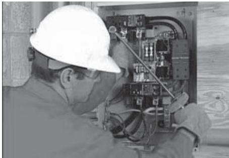
5. Being careful to support the lugs, torque the lugs in the transfer switch to the specifications shown on the transfer switch. Decal located on the inside of the switch door.
