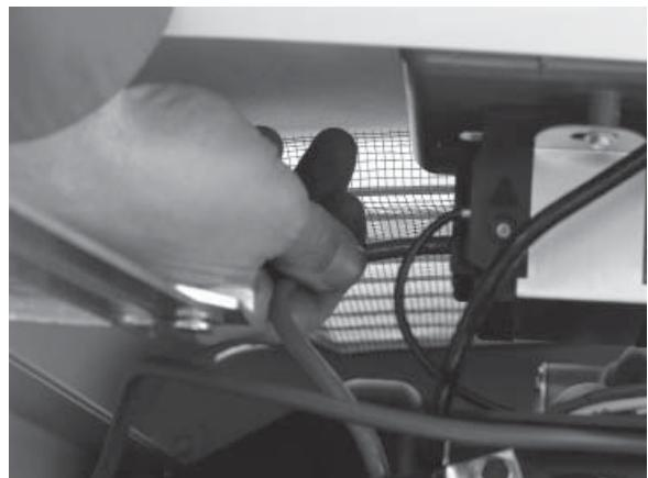
6. Now connect the red and black power leads to the circuit breaker. Since this is a single-phase application, it doesn't matter which wire is connected to which lug.
