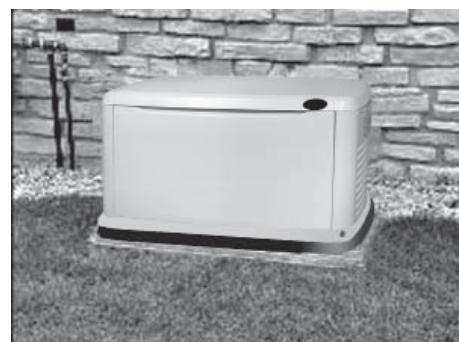
5. Set the generator onto the pad so that the gravel bed extends beyond the generator on all sides. Make sure the generator is level within  $\frac{1}{2}$  inch.
