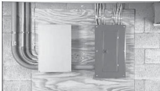
1. If installing the RTSL switch, the service was changed so make sure the terminations are good before re-energizing the utility.
