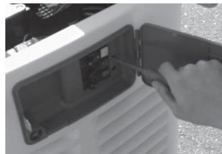
5. Remove the plastic plugs inside the main breaker access area to allow connection of the power leads to the circuit breaker.
