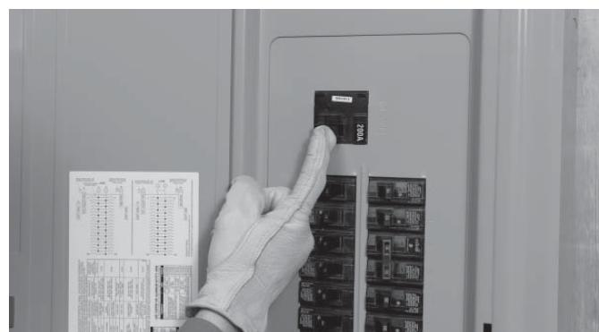
20. Close the main breaker to restore utility power and allow the engine to cool down and shut itself off.
