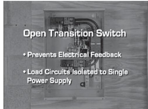
6. The transfer switch being used is an open transition switch. Open transition switches prevent electrical feedback between the generator and the utility by only allowing load circuits to be connected to one power supply at a time.
