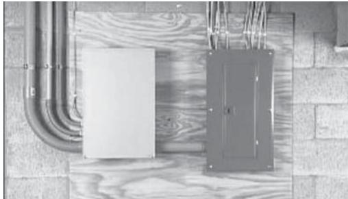
1. Before beginning any installation, make sure power is shut OFF to the main distribution panel and carefully read the Owner's Manual that came with the transfer switch. To simplify the installation process, the transfer switch should be mounted as close to the main distribution panel as possible. Make sure no water or corrosive substances can drip onto the transfer switch enclosure.
