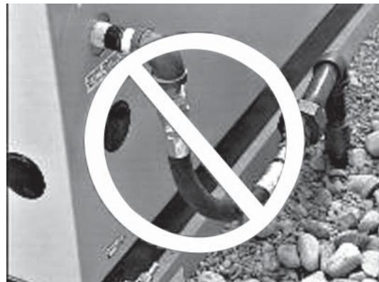
4. Never bend the flexible fuel line to avoid using an elbow. Bending the flexible line decreases its ability to absorb vibrations and defeats its purpose as well as constricts the actual fuel flow.
