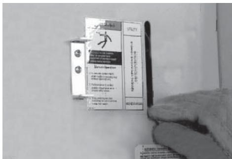
6. Locate the transfer handle, insert the metal end into the slot in the main contactor assembly. Pull the handle DOWN to move the main contacts to the standby power (generator) position. NEVER OPERATE THE TRANSFER SWITCH MANUALLY WHEN LOADS ARE CONNECTED.
