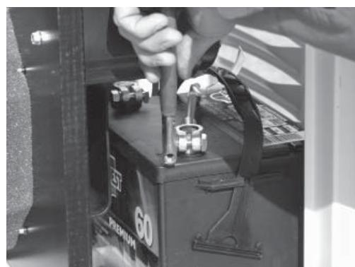
2. Follow all of the procedures and safety precautions in the generator Owner's Manual when installing the battery. Verify the switch is in the off position. When preparing for operational testing, DO NOT connect the battery until transfer switch connections are complete.
