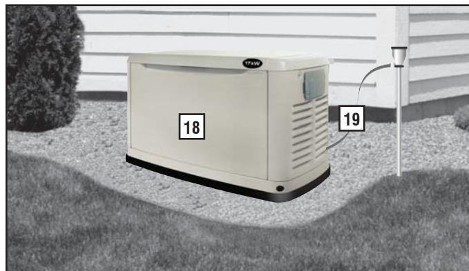
19. Attach one end of the grounding strap (No. 12 AWG stranded copper wire) to grounding rod, and the other end to the grounding lug (located at rear corner of unit). Make sure the grounding rod and strap are not exposed above ground level (NEC code applies to grounding method).
