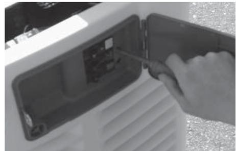
7. Remove the plastic plugs inside the main breaker access area to allow connection of the power leads to the circuit breaker.
