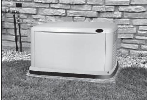
1. Locate the mounting area as close as possible to the transfer switch and fuel supply. Leave adequate room around the area for service access (check local code), and place high enough to keep rising water from reaching the generator. Choose an open space that will provide adequate and unobstructed airflow (see the "Location" section in the Owner's Manual).
