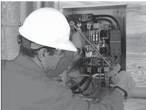
5. Being careful to support the lugs, torque the lugs in the transfer switch to the specifications shown on the transfer switch. Decal located on the inside of the switch door.
