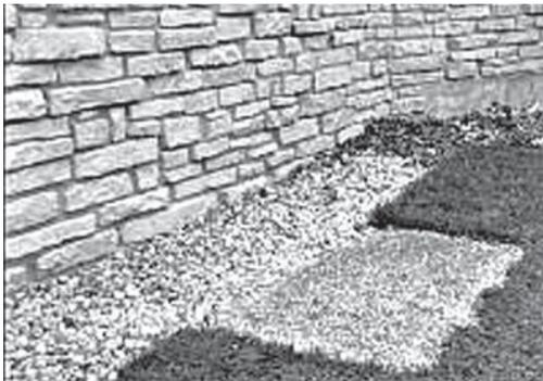
2. Place the unit so air vents won't become clogged with leaves, grass, snow or debris. Make sure exhaust fumes will not enter the building through eaves, windows, ventilation fans or other air intakes. Dig a rectangular area approximately five inches deep and about six inches longer and wider than the footprint of the generator. Cover with polyurethane film and fill with pea gravel or crushed stone. Compact and level the stone. A concrete pad can be poured if desired.
