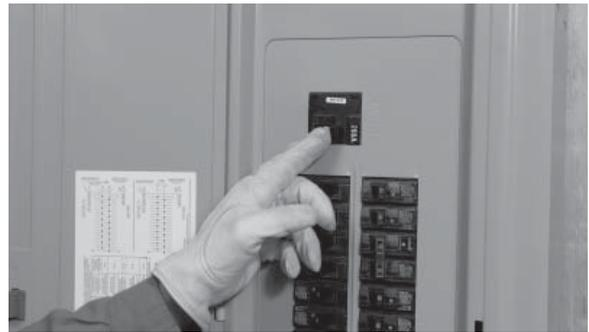
2. Switch the main utility breaker OFF. Refer to NFPA 70-E for the safety equipment required when working inside a live transfer switch.
