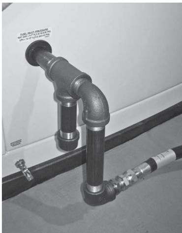
3. When connecting the gas line to the generator, use the provided section of UL Listed or AGA-approved flexible fuel line in accordance with local regulations. The purpose of the flexible fuel line is to ensure that vibration from the generator does not cause a gas leak at one of the connection points, so it's important that the line be installed with as few bends as possible. Installing a sediment trap is also recommended.
