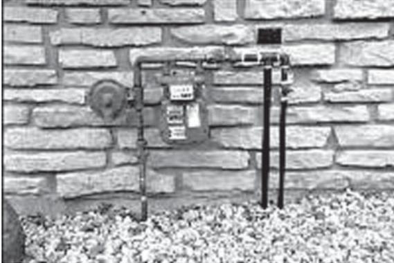
1. Both natural gas and LP Vapor are highly volatile substances, so strict adherence to all safety procedures, codes, standards and regulations is essential. Gas line connections should be made by a certified plumber familiar with local codes. Always use AGA-approved gas pipe and a quality pipe sealant or joint compound. Verify the capacity of the natural gas meter or the LP tank in regards to providing sufficient fuel for both the generator and other operating appliances.
