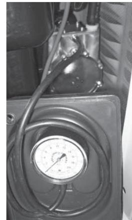
5. After checking for leaks, check the gas pressure at the REGULATOR to make sure there's enough gas pressure for generator operation. **See Owner's Manual for fuel pressure specifications and Btu ratings.** If not within these limits, contact your local gas supplier.
