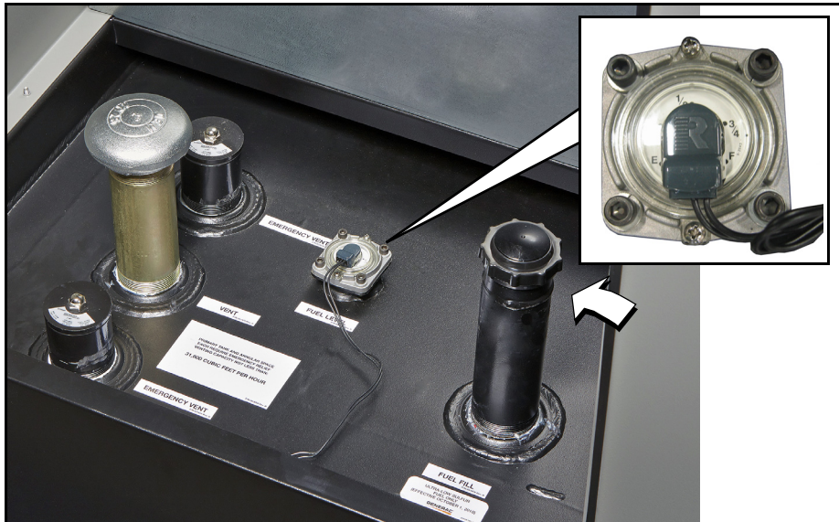
Figure 5-7. Check Fuel Level Gauge and Fill
