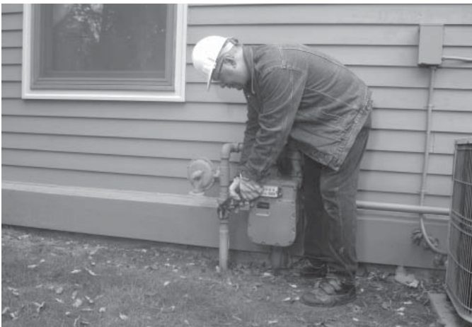
Figure 1.7 — Manual Shutoff Valve
