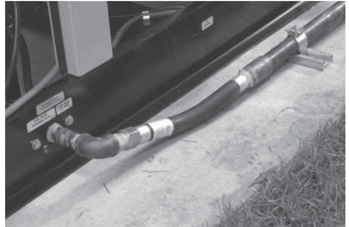
Figure 1.8 — Flexible Fuel Line
