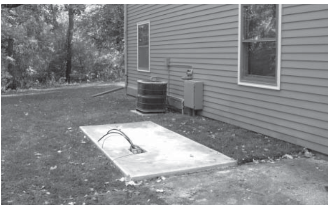
Figure 1.1 — Mounting Pad
