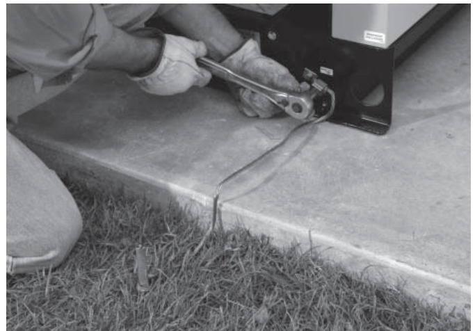
Figure 1.5 — Connect Ground Wire
