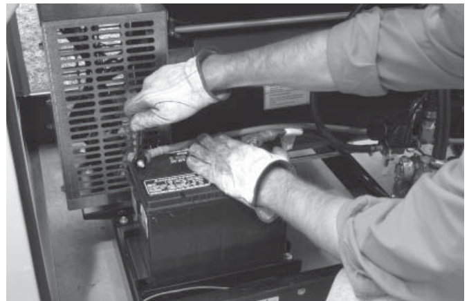
Figure 1.15 — Check Terminal Connections
