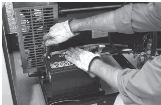
Figura 1.15 — Verifique as conexões do terminal
