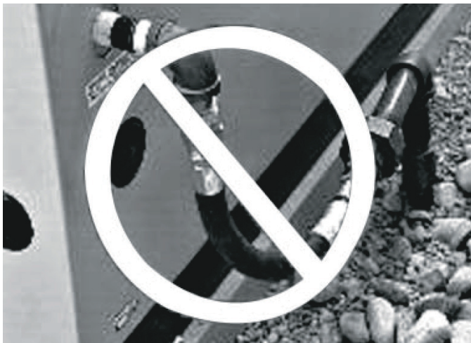
Figure 5-4. Incorrect Routing of Flexible Fuel Line
