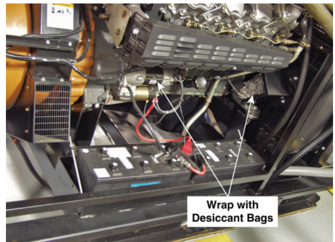
Figure 4 - Wrap with Desiccant Bags
