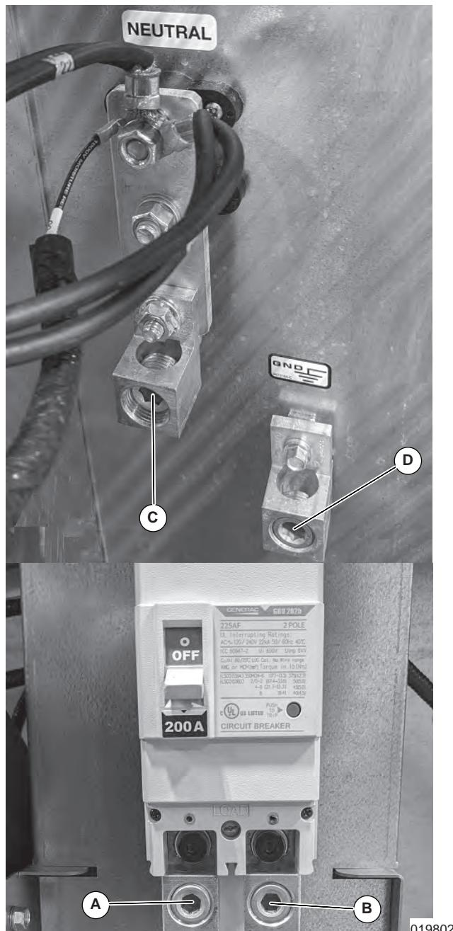
**Figure 5-1. High Voltage 1-Phase Connections**
