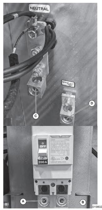
Figure 5-1. High Voltage 1-Phase Connections
